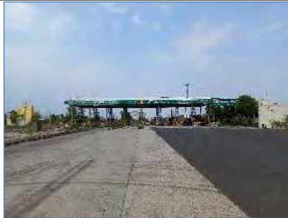
Toll Plaza at km 92+500
