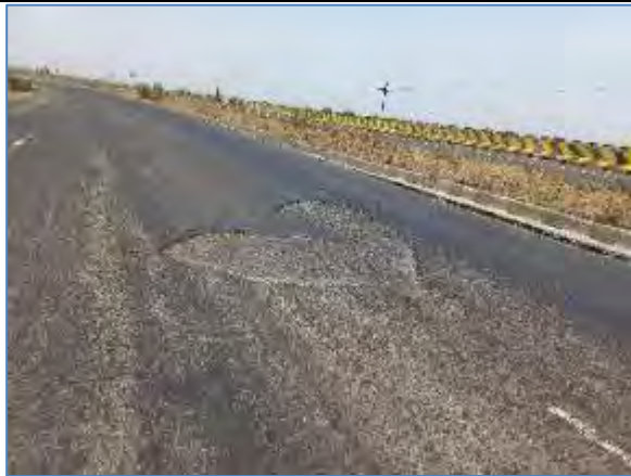
Delimitation at km 100.050-LHS
