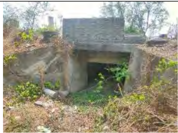
Slab Culvert at Km 51+180
