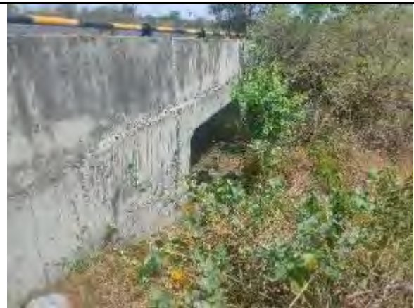
Box Culvert at Km 83+092
