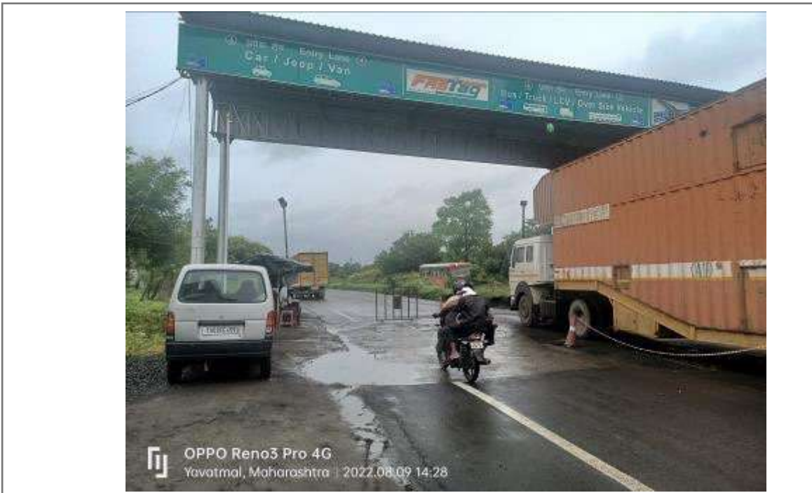
Photo 9: Electronic Toll Collection (ETC) lane
