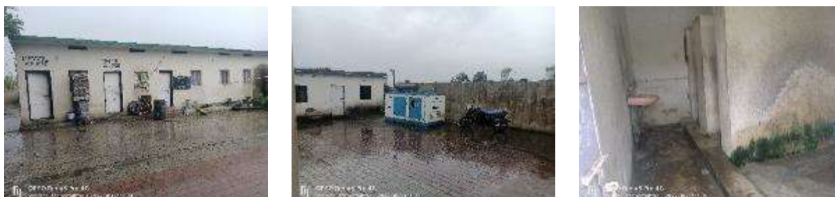
Figure 2-4. Facilities at Darodha Toll Plaza
