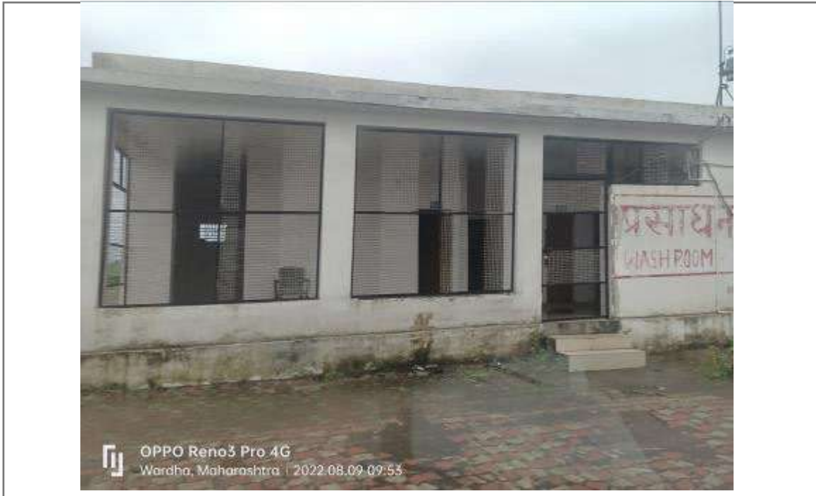
Photo 7: Washroom facility on the toll plaza
