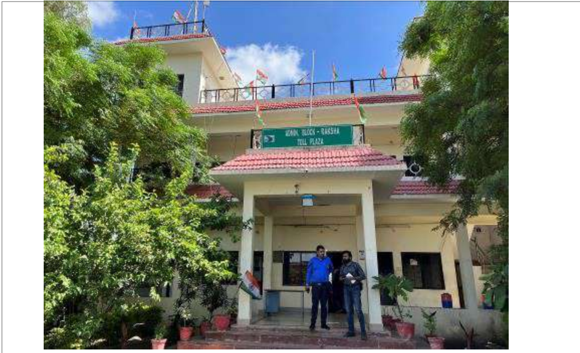
Photo 1: Toll plaza building
