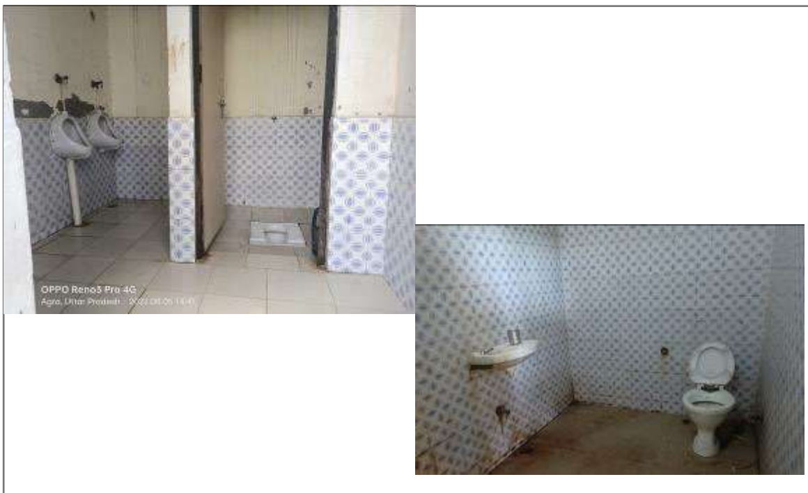
Photo 6: Toilet facilities at the toll plaza
