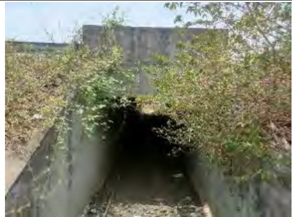
Box Culvert at Km 42+387
