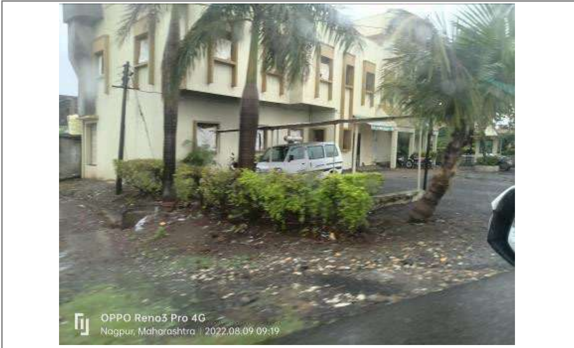
Photo 1: Toll plaza building
