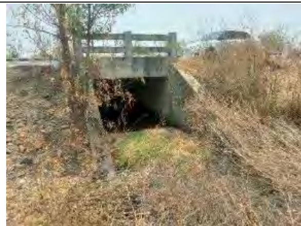
Slab Culvert at Km 46+847
