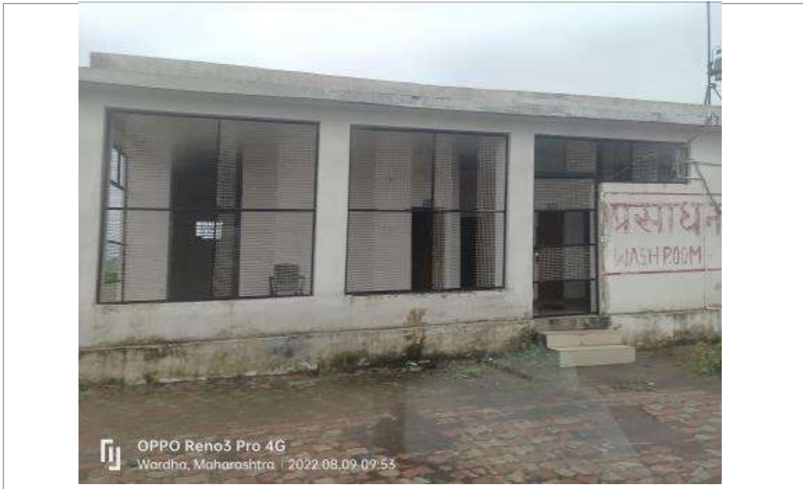
Photo 7: Washroom facility on the toll plaza
