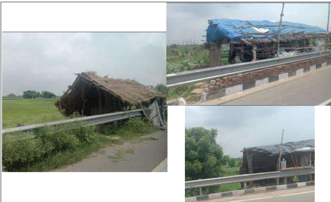
Photo 2: Encroachments in the ROW
