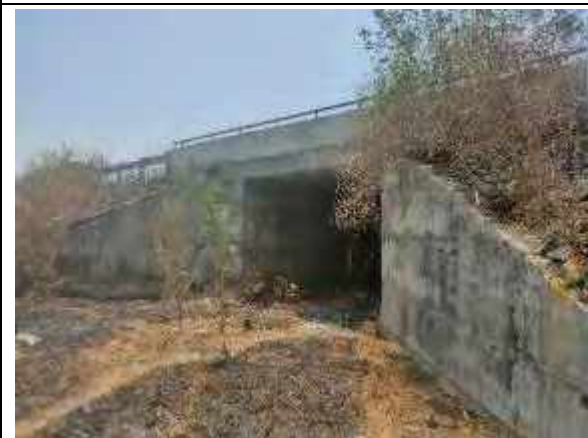
Box Culvert at Km 93+985
