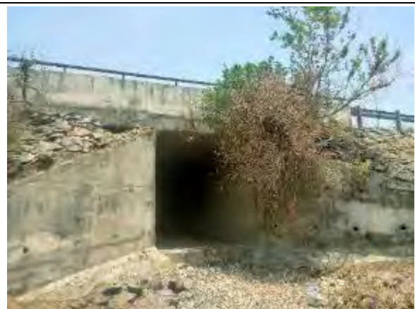
Box Culvert at Km 95+914
