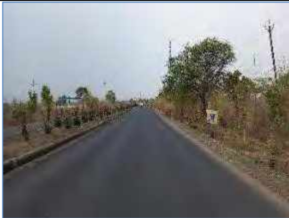
Fair condition km 88.000-LHS
