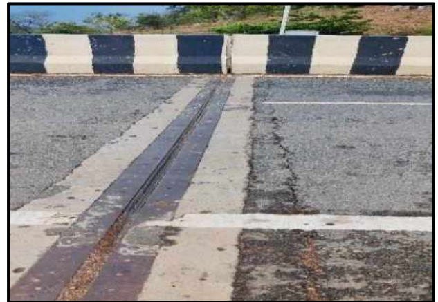
Major Bridge at Ch. 1319+870
