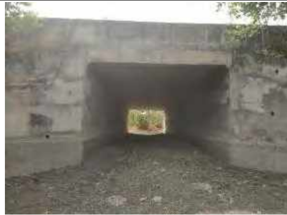
Box Culvert at Km 130+662
