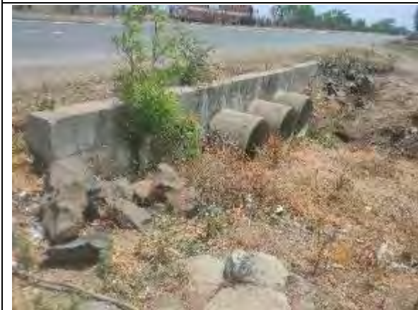
Pipe Culvert at Km 90+720
