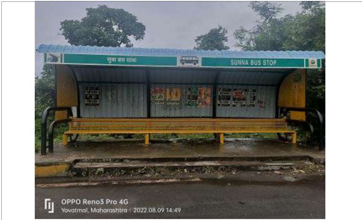
Photo 10: Bus stop along National highway
