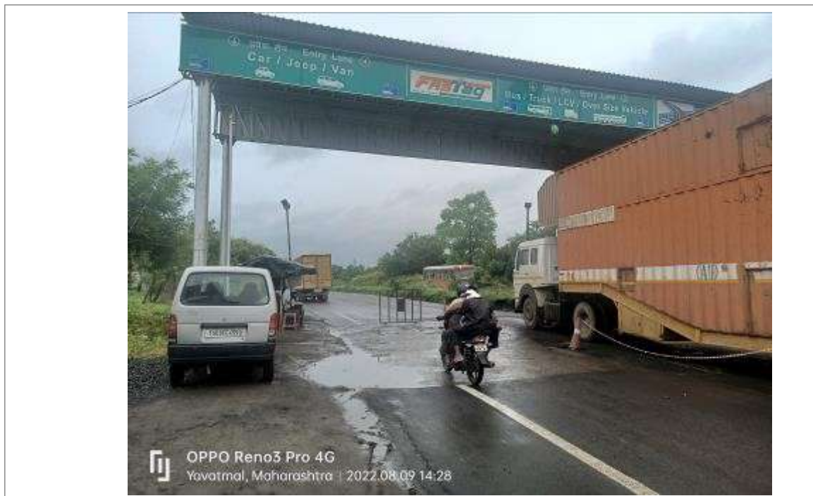
Photo 9: Electronic Toll Collection (ETC) lane
