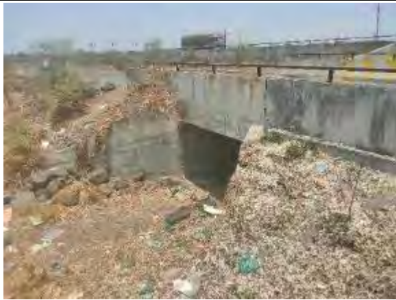
Box Culvert at Km 100+121
