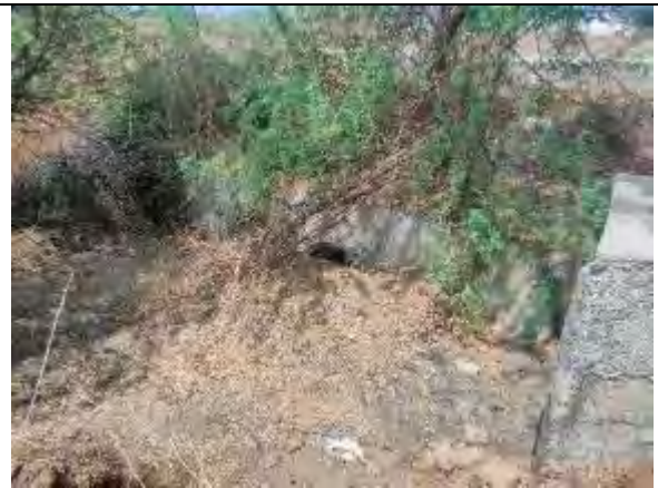
Pipe Culvert at Km 105+494
