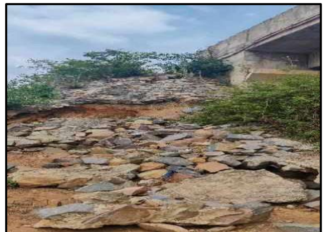
Major Bridge at Ch. 1356+285
