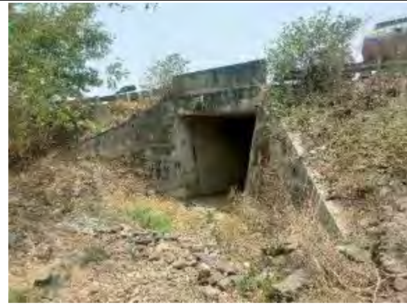
Slab Culvert at Km 42+335
