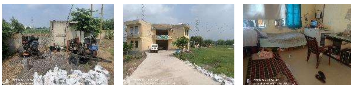
Figure 2-4. Facilities at Raibha Toll Plaza
