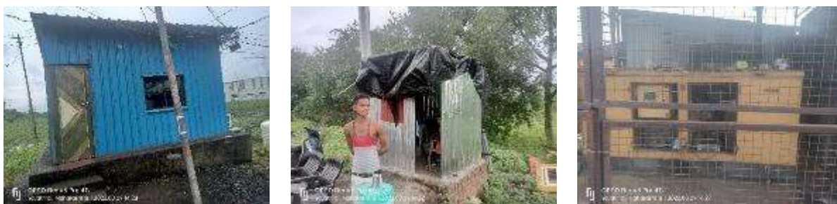
Figure 2-5. Kelapur Toll Plaza
