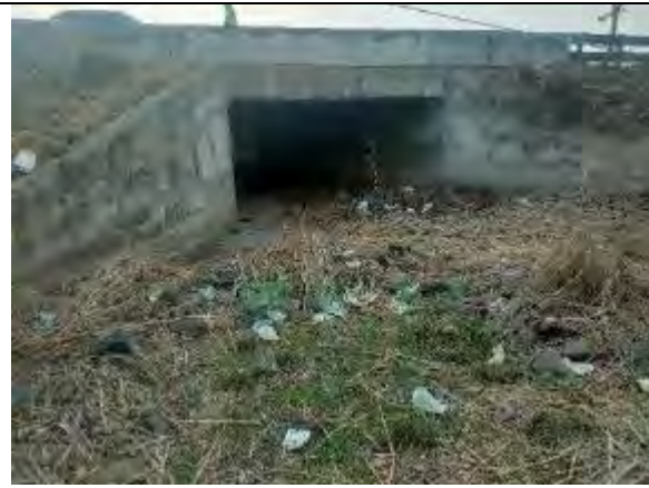
Box Culvert at Km 141+925
