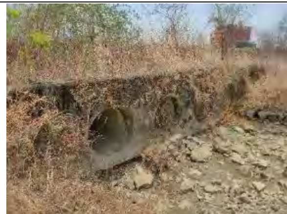
Pipe Culvert at Km 40+262
