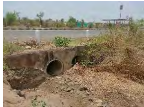
Pipe Culvert at Km 38+483
