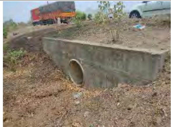
Pipe Culvert at Km 39+249
