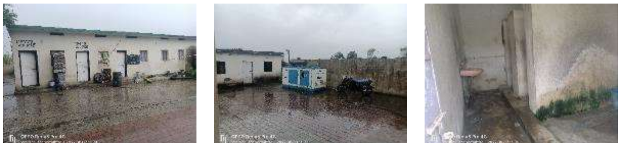
Figure 2-4. Facilities at Darodha Toll Plaza
