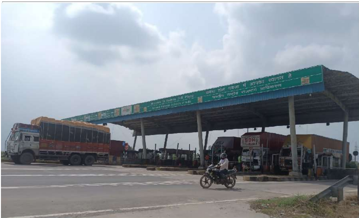
Photo 8: Raibha Toll plaza
