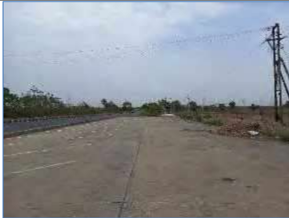
Truck Lay bye on LHS km 68.240
