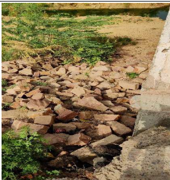
MNBR at CH. 31+547
