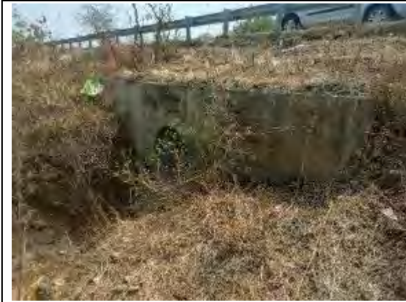
Pipe Culvert at Km 122+122
