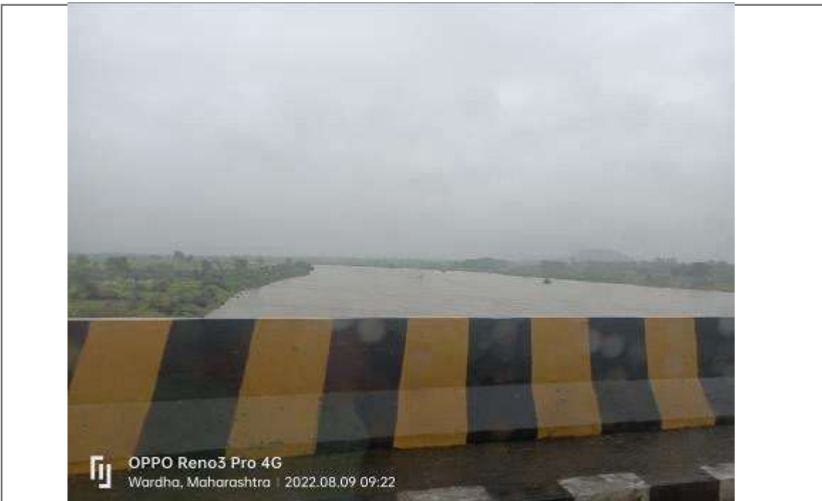
Photo 2: Bridge over the river in project area
