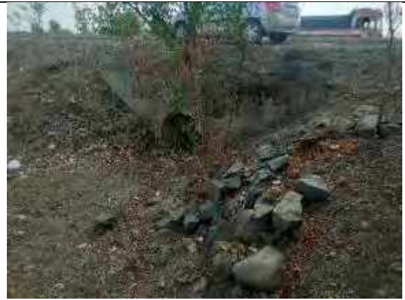
Pipe Culvert at Km 135+596
