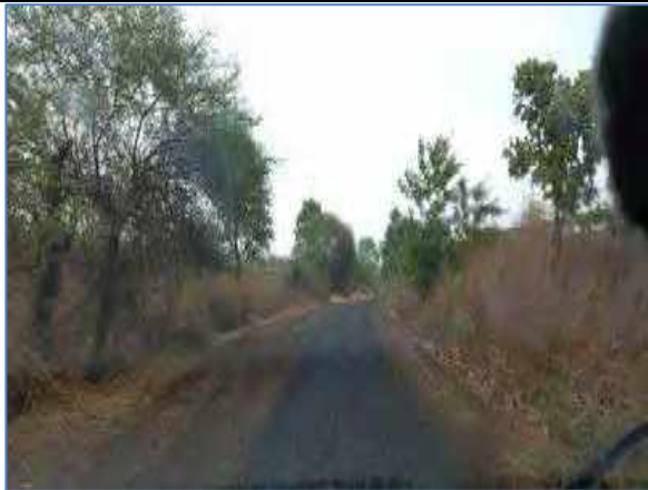
Service Road @ km 128.800 to km 129.150 - LHS_5.80m wide
