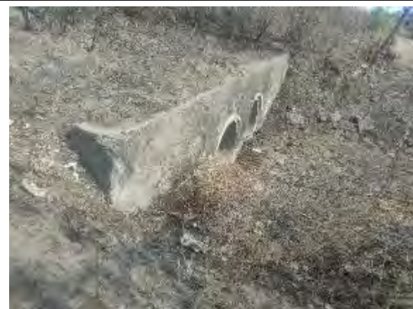
Pipe Culvert at Km 61+789
