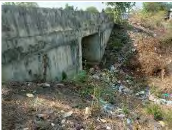
Box Culvert at Km 134+395
