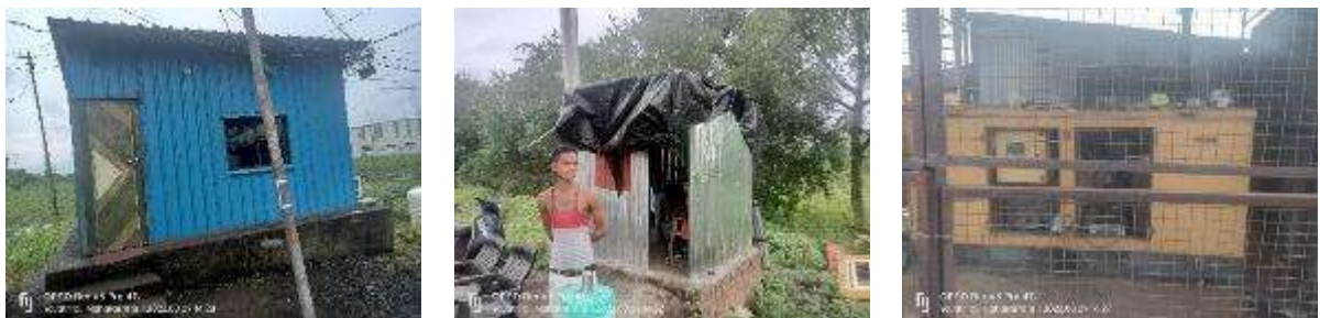
Figure 2-5. Kelapur Toll Plaza
