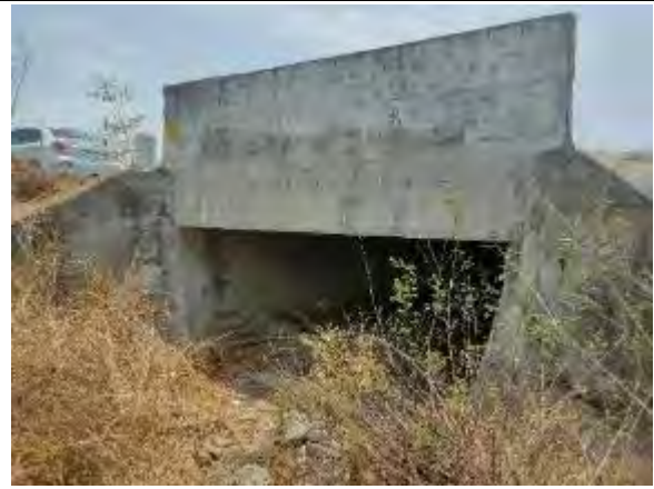
Slab Culvert at Km 45+985
