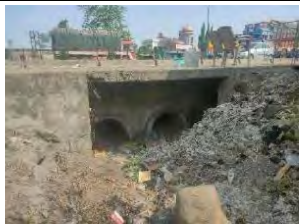
Pipe Culvert at Km 63+168
