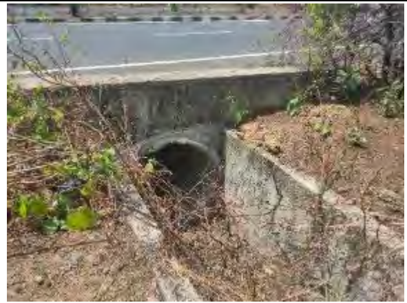
Pipe Culvert at Km 125+615
