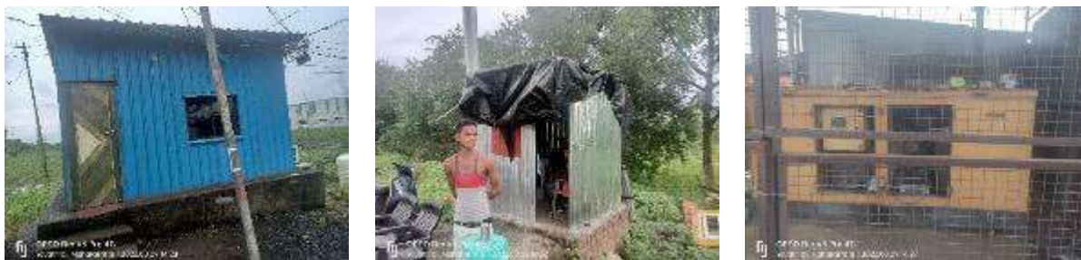
Figure 2-5. Kelapur Toll Plaza
