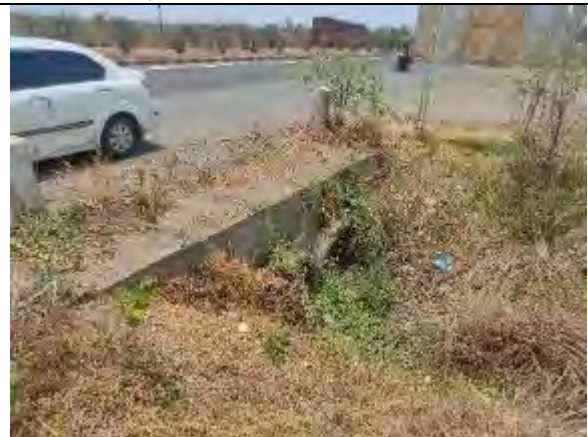
Pipe Culvert at Km 43+166
