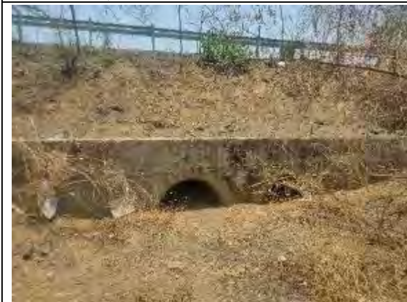
Pipe Culvert at Km 111+349
