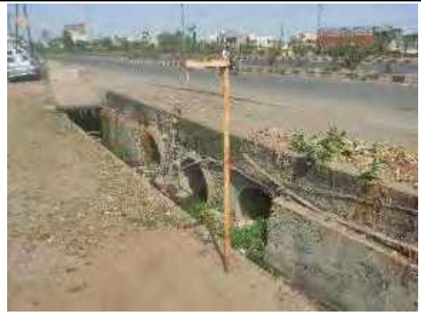
Pipe Culvert at Km 73+785
