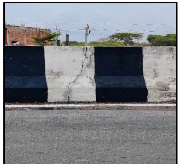
MINOR BRIDGE AT 1359+451
