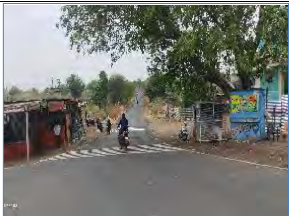
Major Junction at km 153.204 RHS
