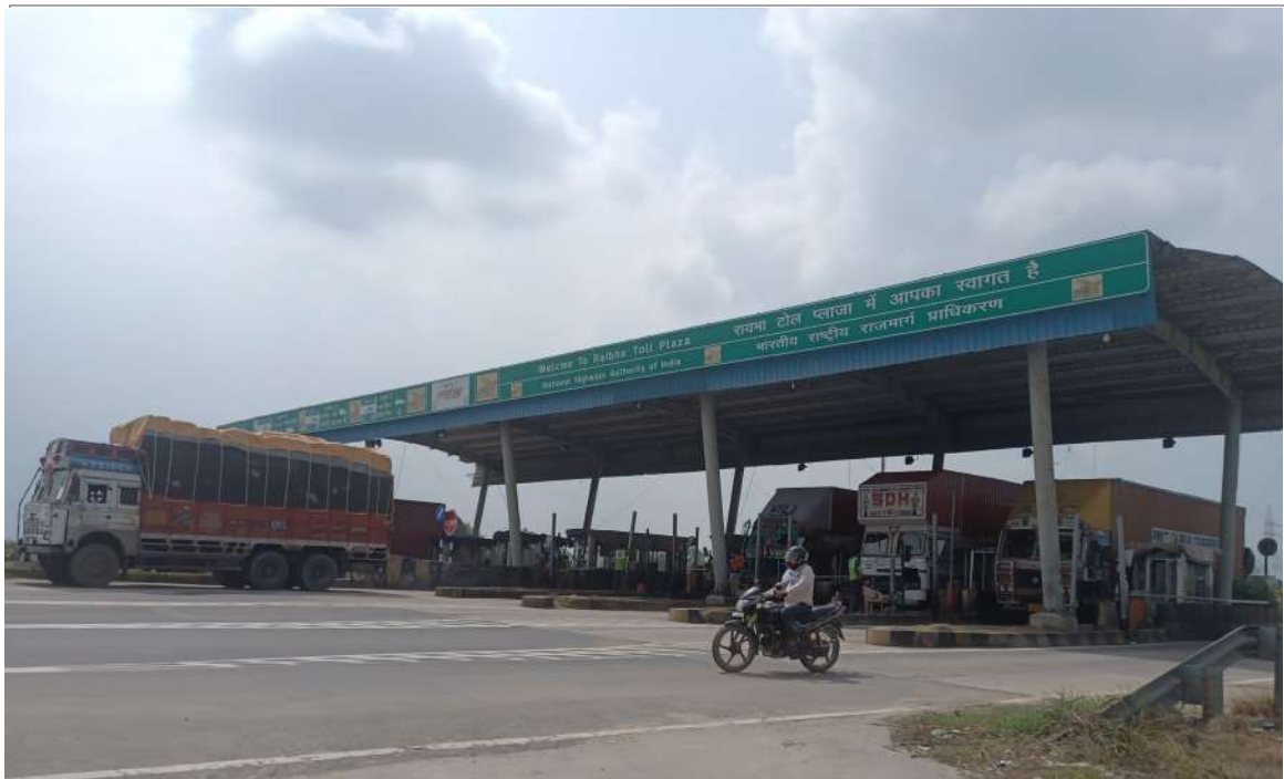
Photo 8: Raibha Toll plaza
