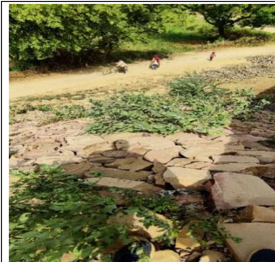
MNBR at CH. 17+661
