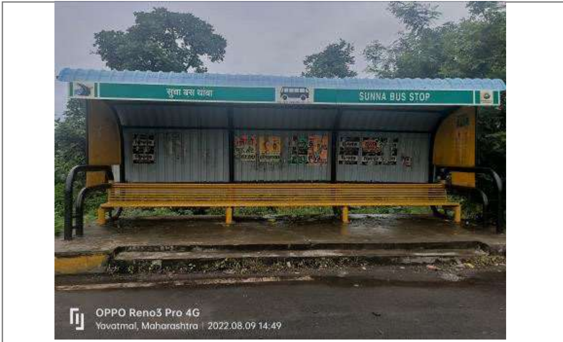
Photo 10: Bus stop along National highway
