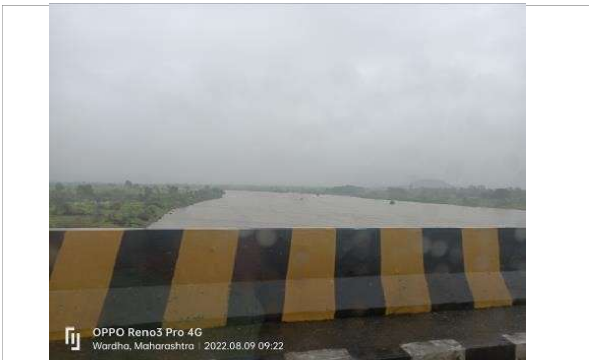
Photo 2: Bridge over the river in project area
