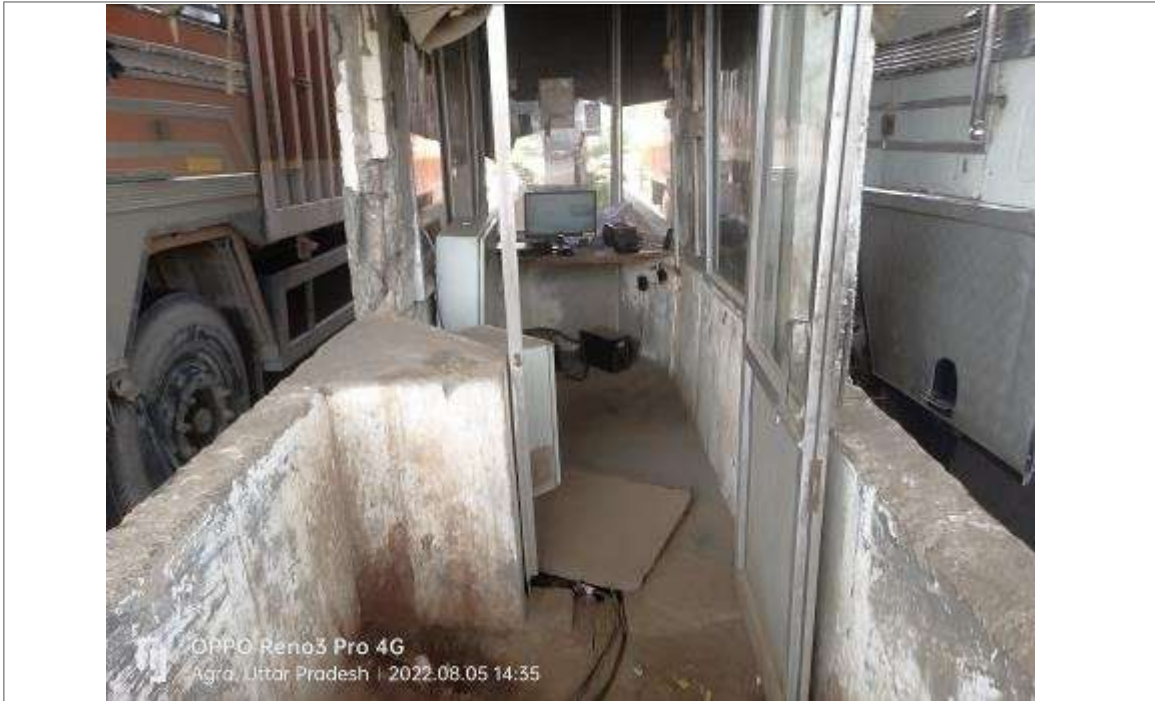
Photo 9: Inside view of toll booth
