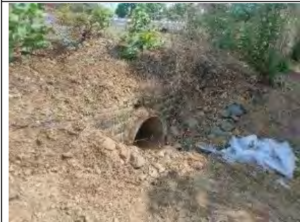
Pipe Culvert at Km 127+180
