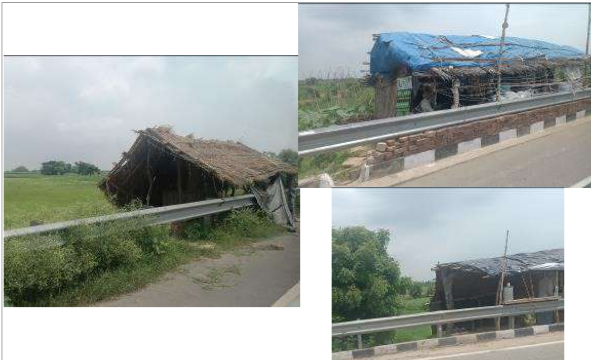
Photo 2: Encroachments in the ROW
