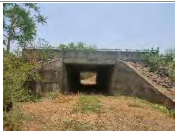
Slab Culvert at Km 164+145
