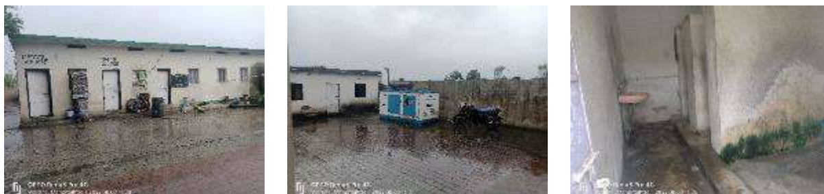
Figure 2-4. Facilities at Darodha Toll Plaza
