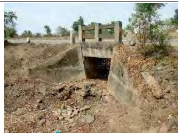
Slab Culvert at Km 57+155
