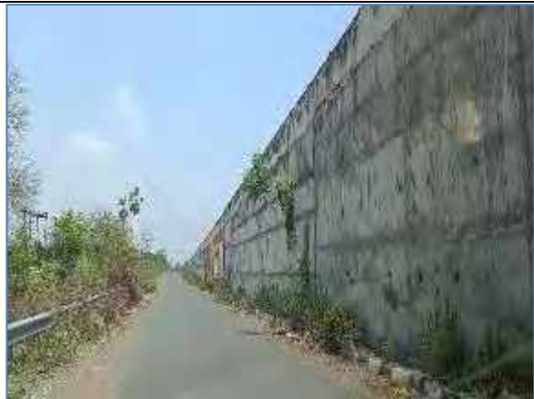
Service Road @ km 66.700 to km 67.350-LHS_5.5m wide
