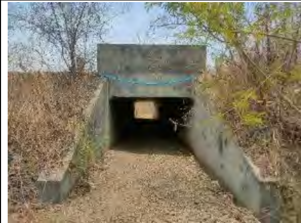
Box Culvert at Km 41+016
