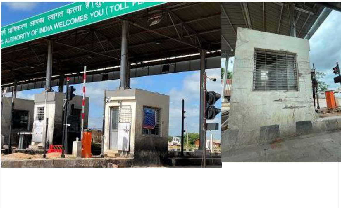
Photo 2: Electronic Toll Collection (ETC) lanes and toll booths at the toll plaza
