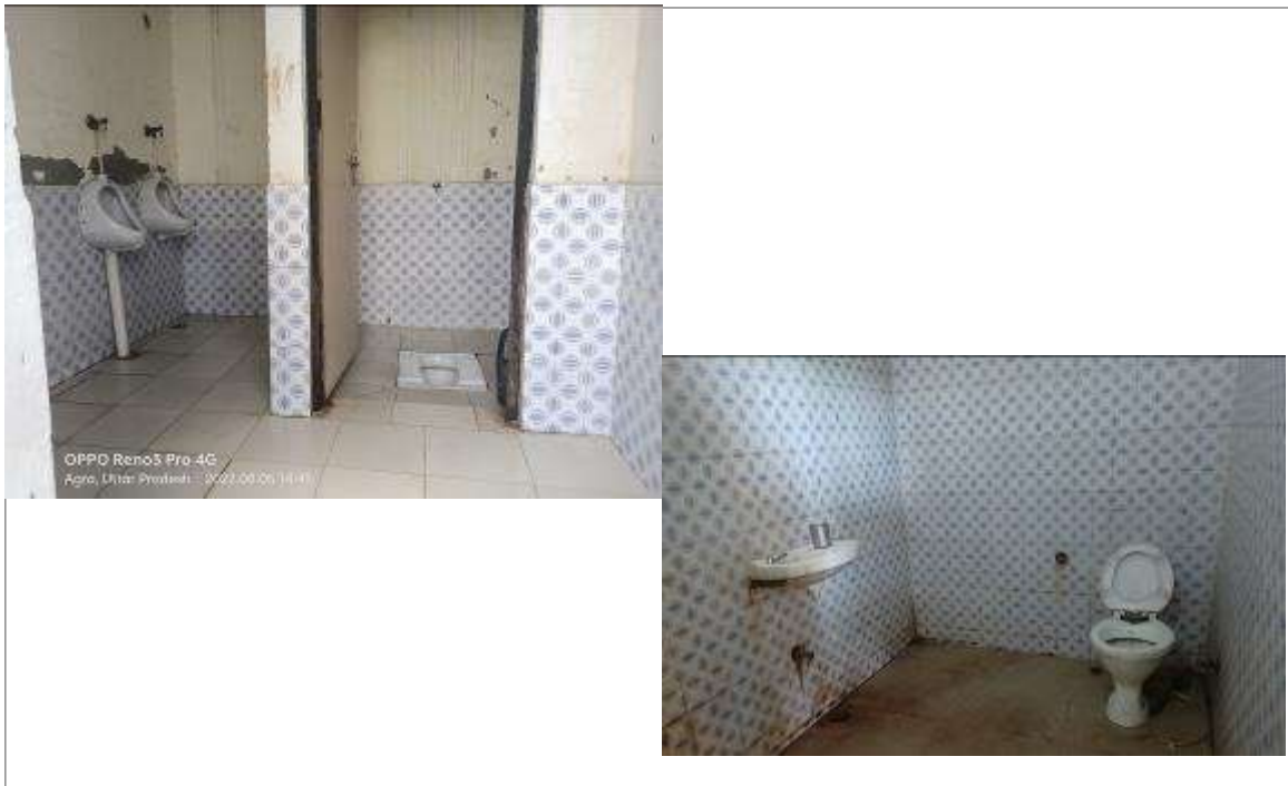
Photo 6: Toilet facilities at the toll plaza
