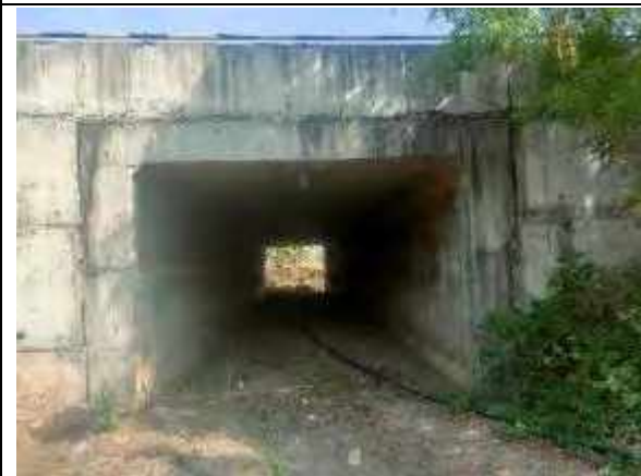
Box Culvert at Km 66+244
