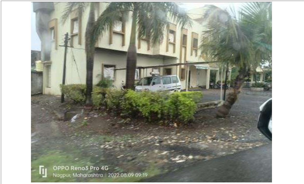
Photo 1: Toll plaza building
