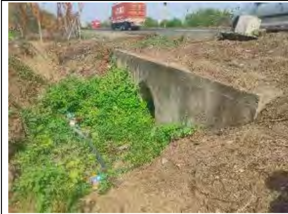
Pipe Culvert at Km 70+605
