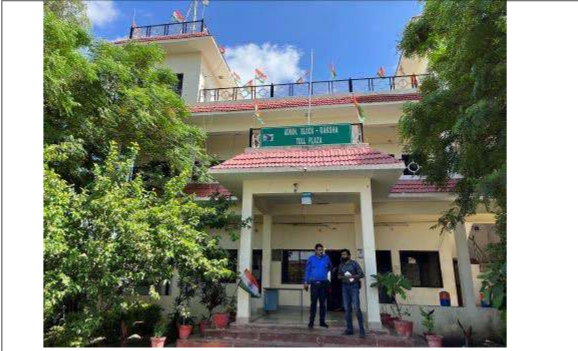
Photo 1: Toll plaza building
