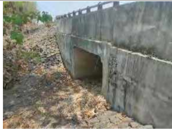
Box Culvert at Km 161+580
